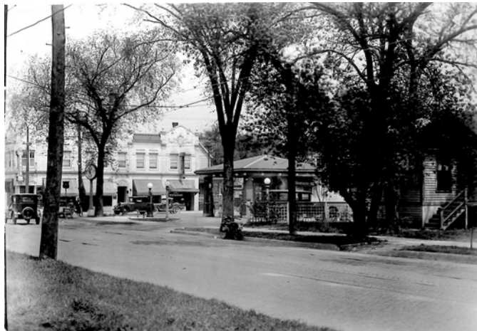
Late 1920s view along Harlem north toward Chicago Avenue, showing the roadway with its new brick surface along this stretch.
