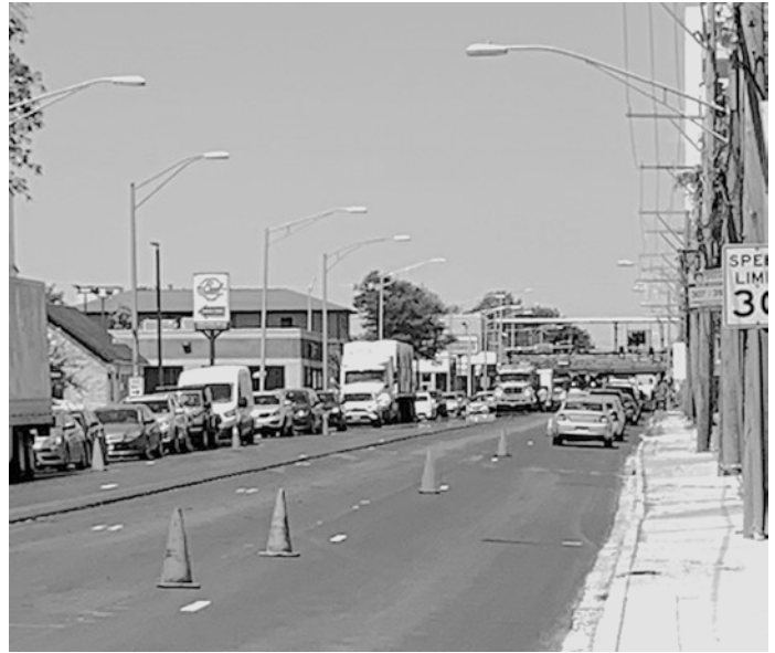
Harlem Avenue. June 2022. Construction (and congestion) continues.
