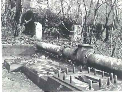
Are these pipes remains of the CCC camp?
